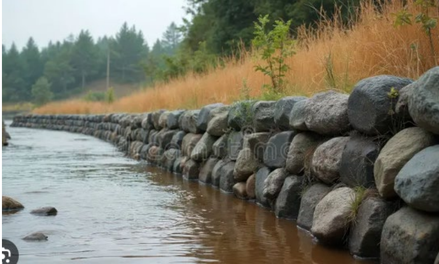
Figure 2 Example of Rock stabilisation of riverbank
