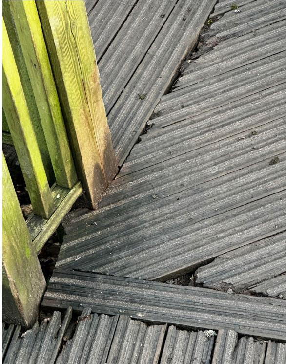
Figure 2 - Examples of wood reaching the end of its life
