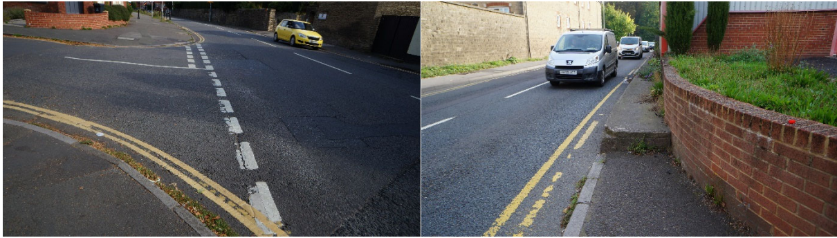
Figure 6-10: Example of flared side-road junction with no tactile information (left) and example of narrow and abruptly ending footway on a busy road (right)
