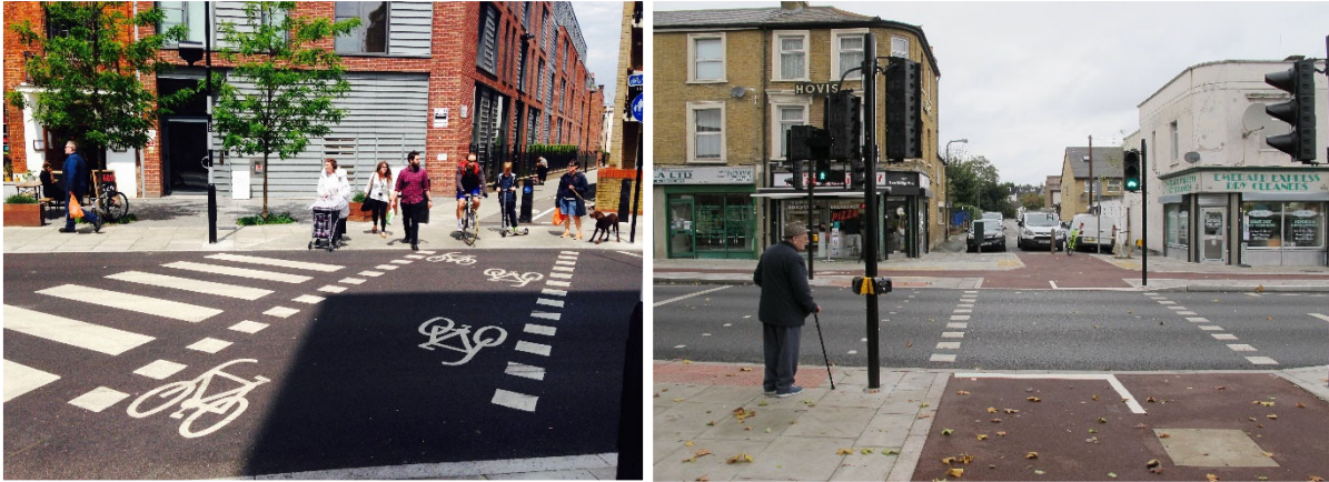
Figure 6-11: Richmond Road Parallel Crossing (Left) and Lea Bridge Road, Parallel Ped/Cycle Crossing (Right)
