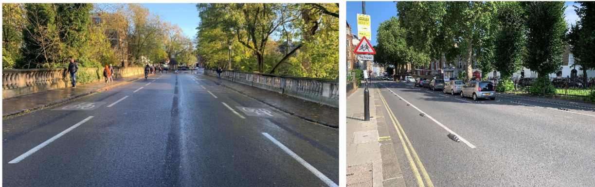
Figure 6-13: Wide ‘Dutch Style’ advisory cycle Lanes Magdalen Bridge, Oxford (left) and light segregation on Royal College Street, Camden (right)
