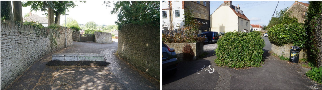
Figure 6-16: Examples of existing modal filters in Frome (Spring Lane, left and Lower Keyford, right)
