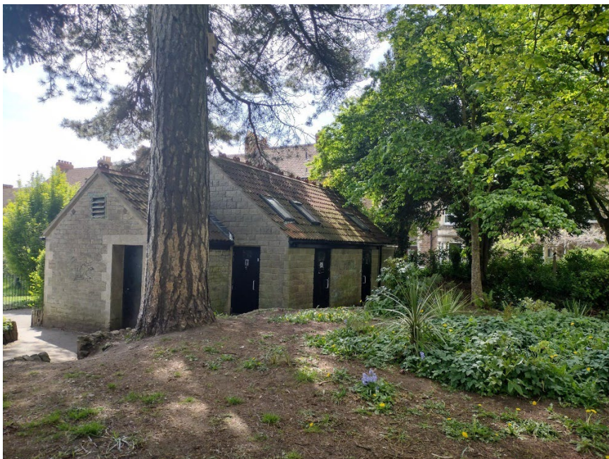
Current toilet block
