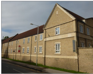
FIGURE 12. OFFICE BUILDINGS IN FRO
