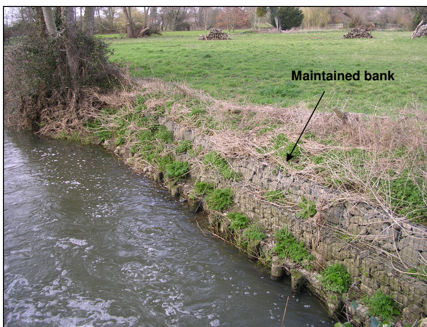
Photo 4.2 – Maintained bank at Baltonsborough along the Baltonsborough Millstream
