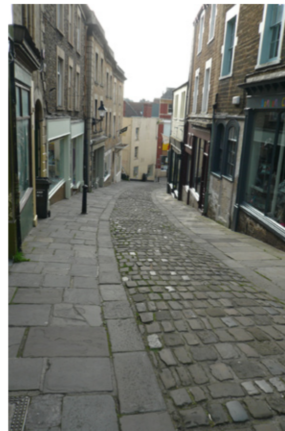
Reclaimed Pennant Stone slabs and setts, Catherine Hill
