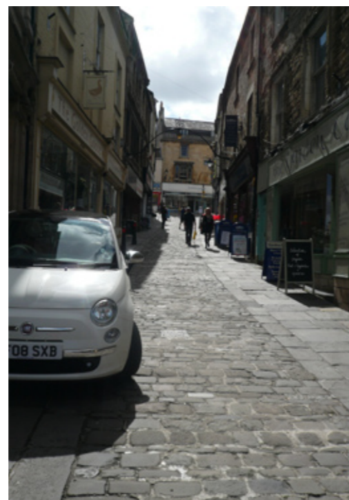
Stony Street : reclaimed pennant slabs and setts
