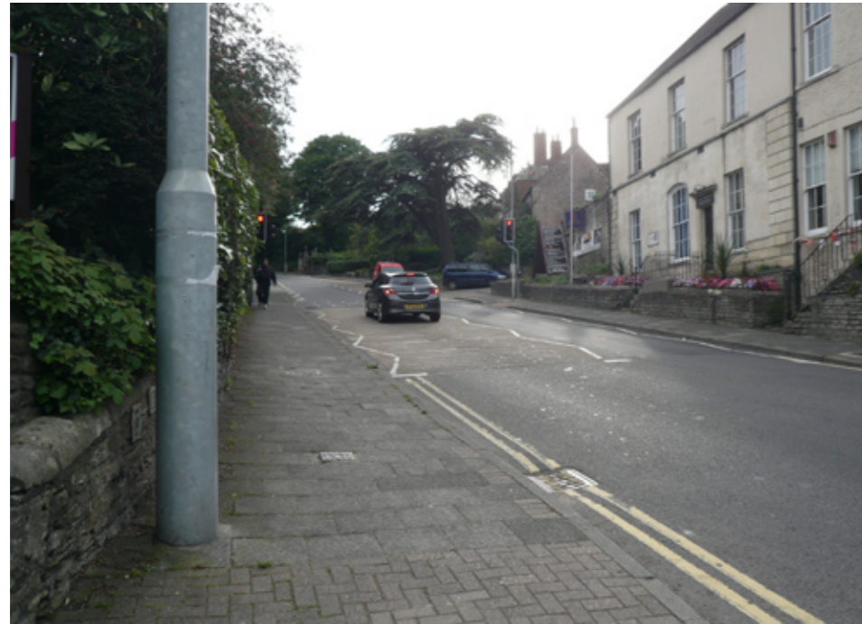
Existing : Bath Street carriageway
