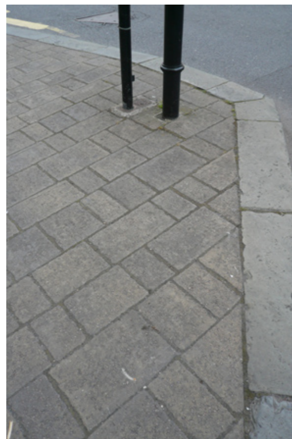
Pre-cast Concrete Blocks with reclaimed stone kerb
