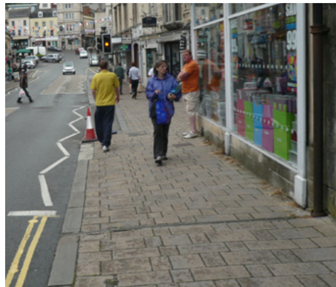
Pre-cast Concrete Blocks and kerbs : The Bridge
