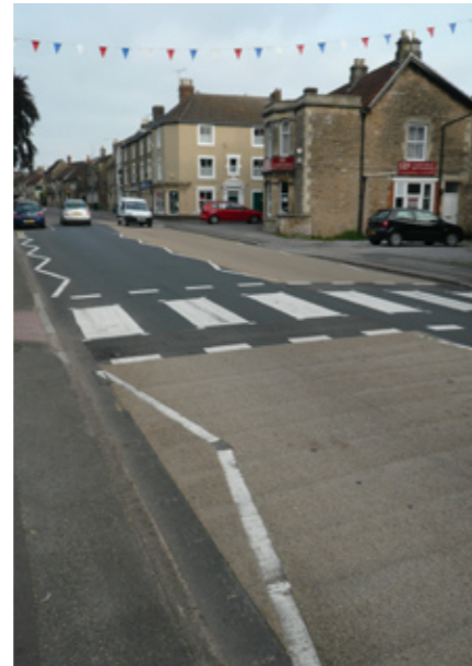
In-situ : resin bonded gravel over bitmac
