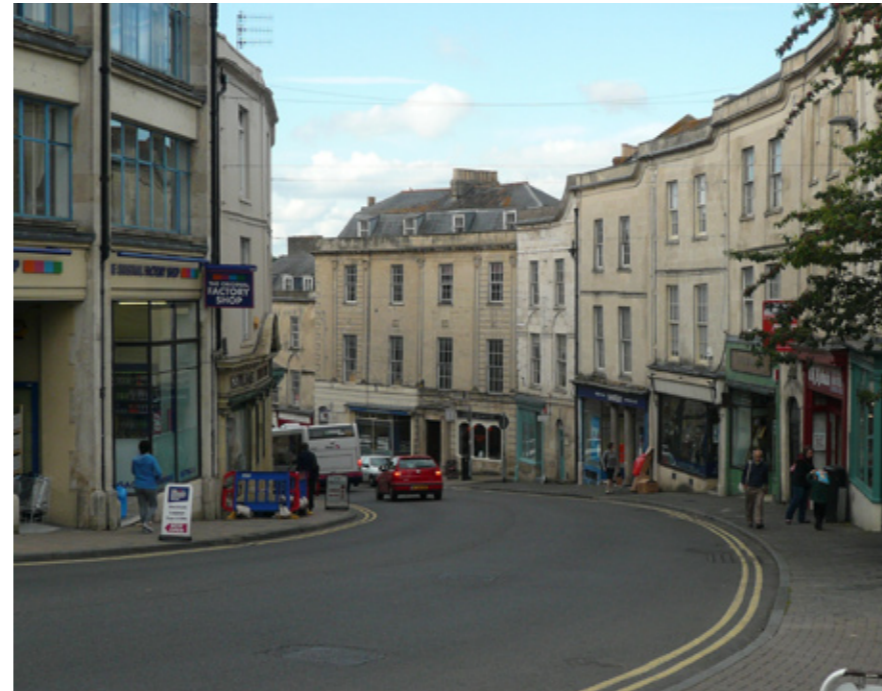
Existing : Bath Street carriageway
