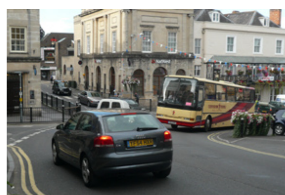
Wide carriageway - designed as a trunk road
